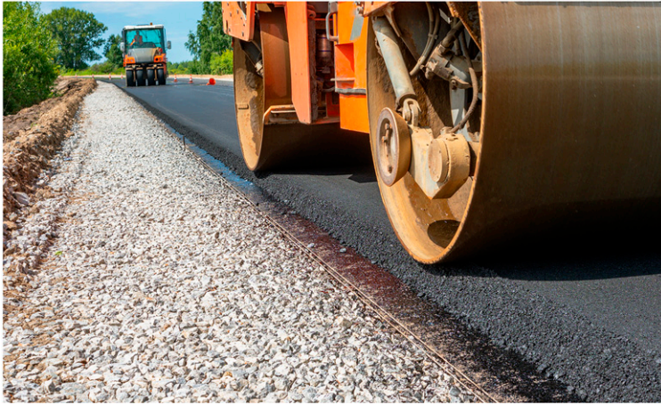
One way to improve road sustainability is to find substitutes for the traditional building blocks of pavement's foundations, such as limestone aggregate. Image credit: Shutterstock/Andrei Ksenzhuk.
